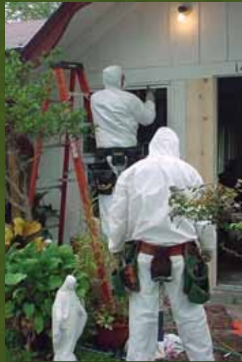
Contractors install new energy efficient windows
