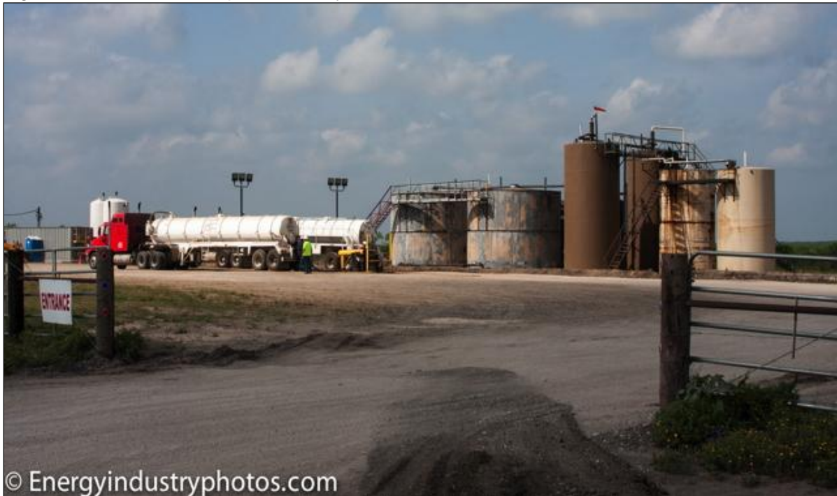
Figure 7-4: Saltwater Disposal Facility North of Tilden Texas 399
