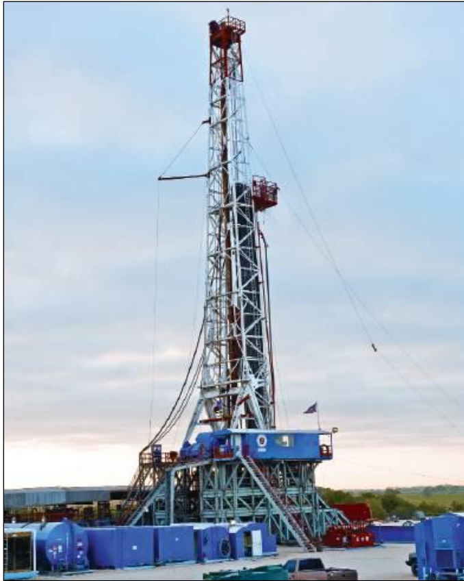
Figure 4-2: Magnum Hunter Resources Drilling Rig in the Eagle Ford
