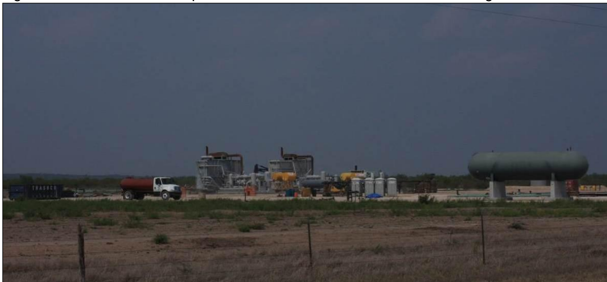
Figure 7-1: Natural Gas Compressor Station under Construction in the Eagle Ford Shale
