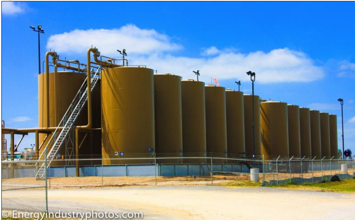
Figure 7-3: Centralized Tank Battery in Gonzales County 397
