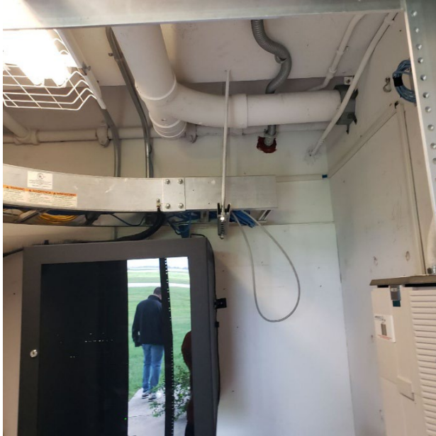
Comm Room North Interior Wall
