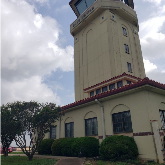
West Exterior Wall
